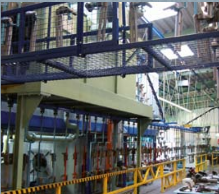
Powder coating unit
